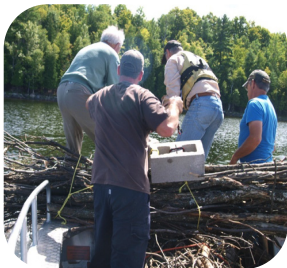
Figure 7: Tying an anchor to a brush pile and depositing it into the lake.
