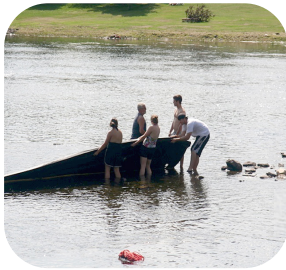
Figure 5: Installing the silt curtain around the work site.
