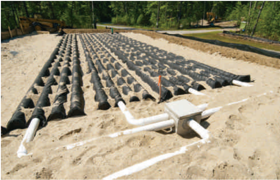
Photos: Cataraqui Region Conservation Authority
