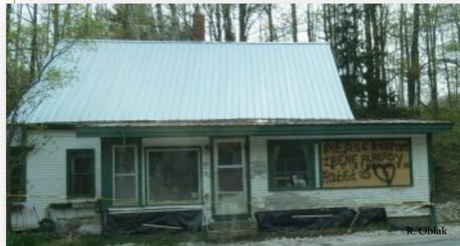
Home damaged by flood near Killington, Vermont
