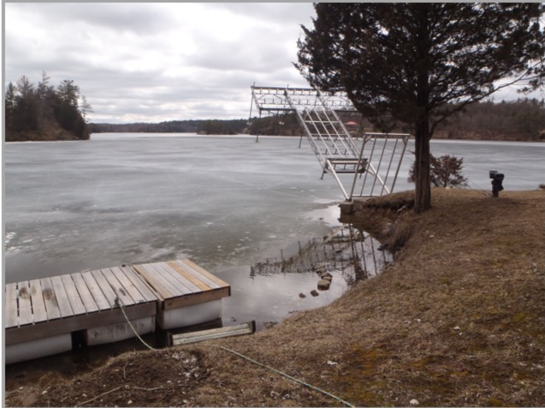
PROPERTY B - Photo 3 – Shoreline erosion with no buffer
