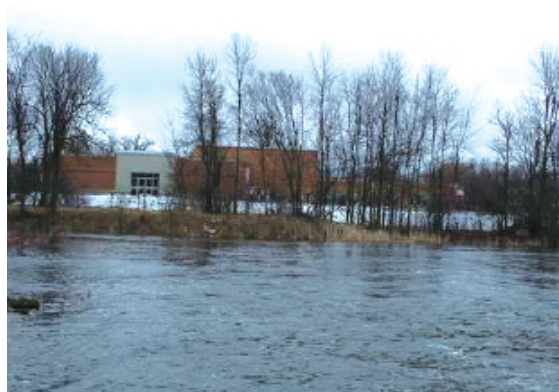
Perth Water Treatment Plant
