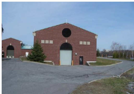
Lemieux Island Water Purification Plant
